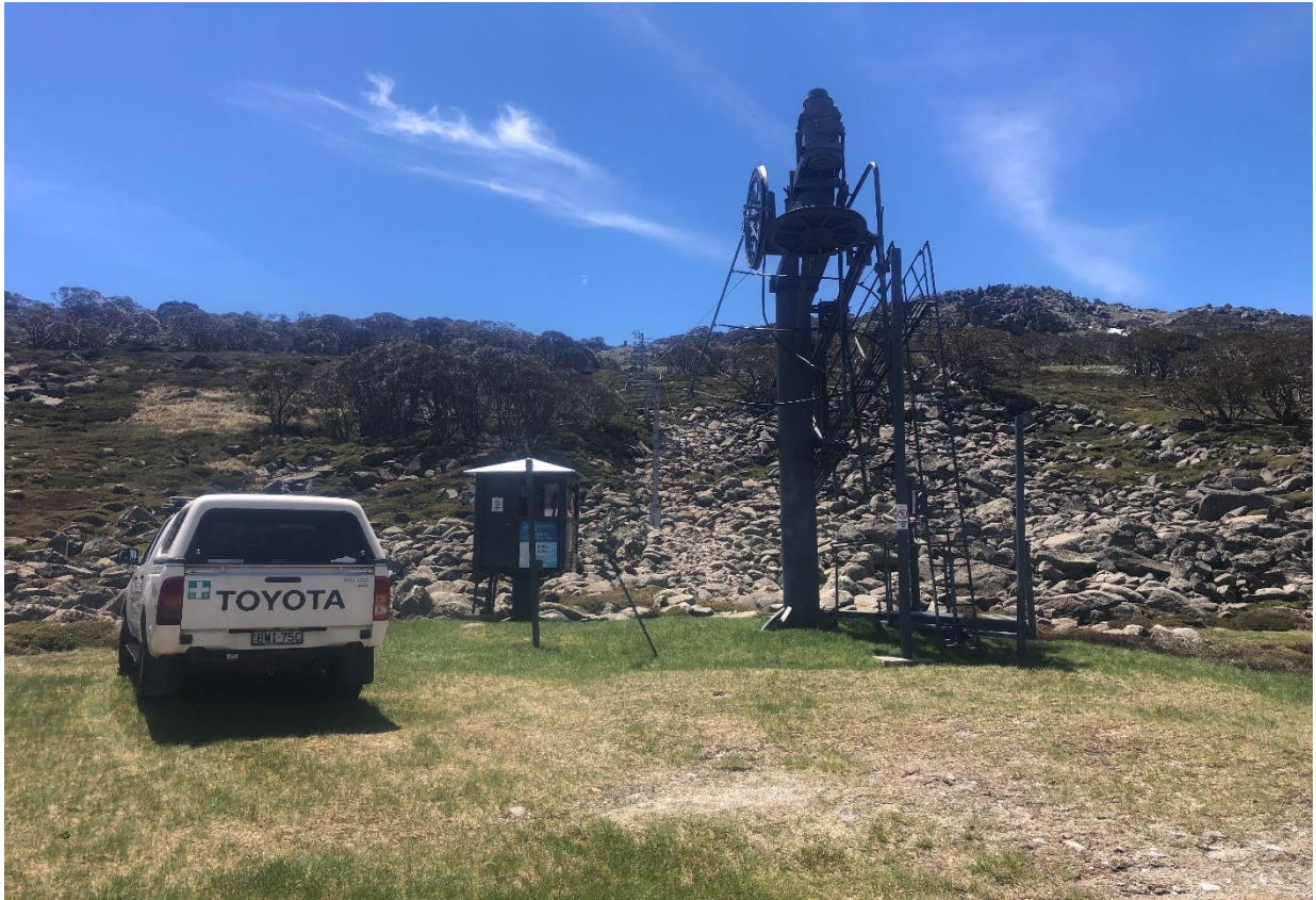
Photo 1: The proposed chairlift will be located on the existing alignment of the Guthries Poma and will take advantage of the existing disturbed area for the chairlift bottom station and Tower 1. Tower 2 will be located above the boulderfield, which is a key habitat for the Mountain Pygmy-possum, enabling the removal of the existing Tower 1, which is located within the boulderfield.
